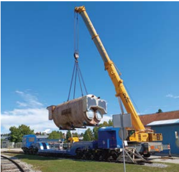
Loos steam boiler
