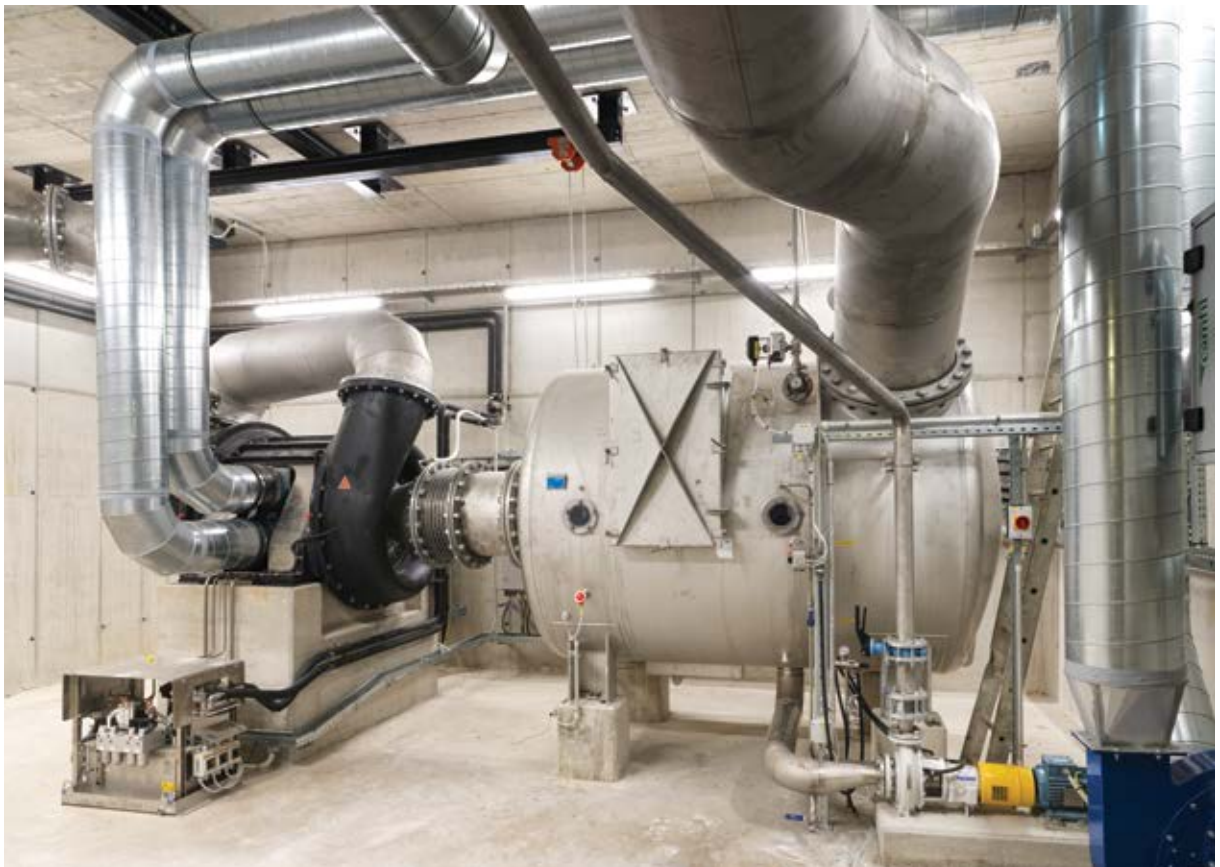
New RunEco vacuum system by Runtech, including EP600 turbo blower and EcoDrop and EcoSep water separators
