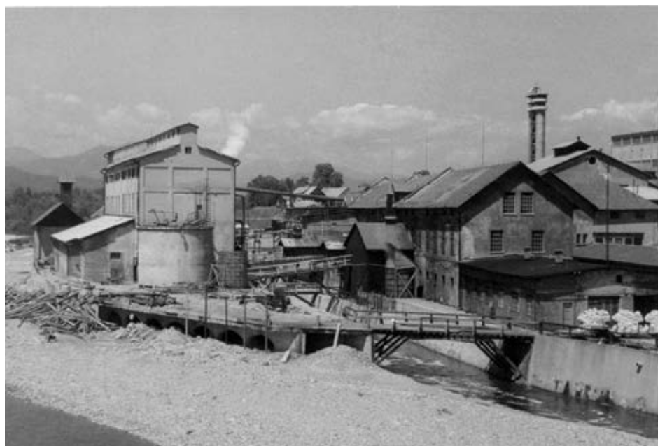
A view of the old section of the pulp mill on an island in the Sora River in 1964.
